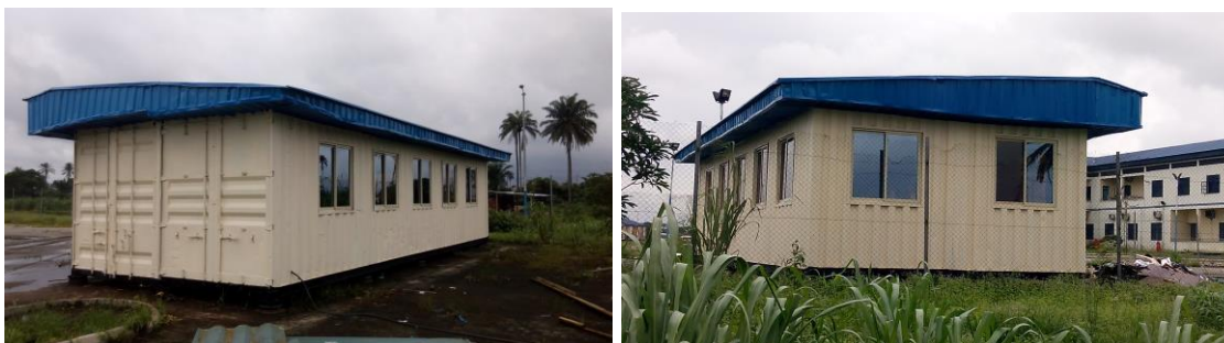
Figure 1: Department of Earth Sciences laboratory built from two shipping containers
